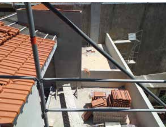
Figure 9. Terraces are ongoing
