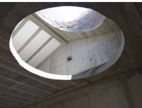
Figure 11. Roof insulation is almost completed
